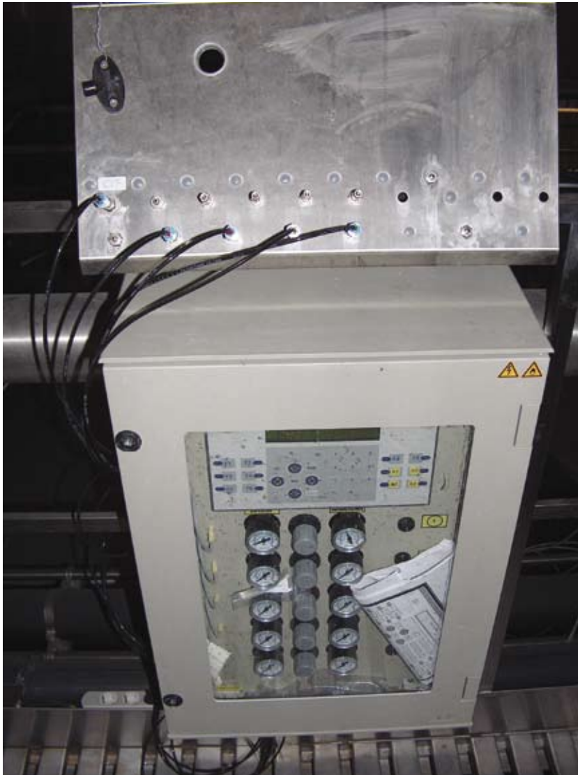
Control panel for a microoxygenation device at Falua winery, Ribatejo, Portugal.
